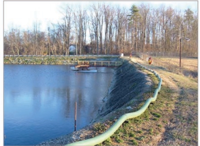
Vapor Distribution Line installed around Lagoon
