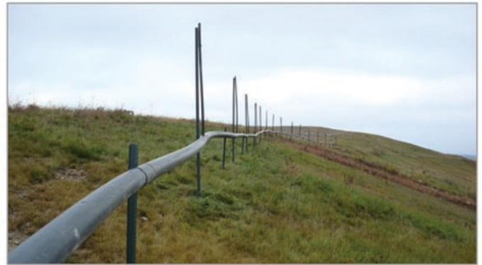
Stanchions Mounted on Temporary Posts
