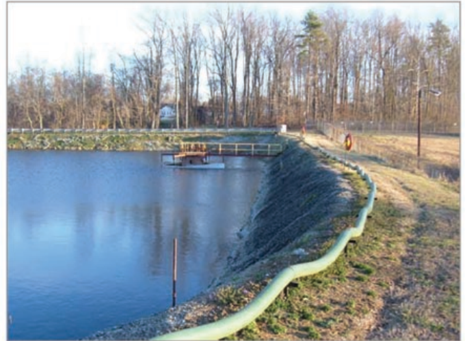
Vapor Distribution Line installed around Lagoon
