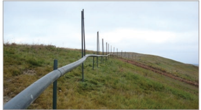
Stanchions Mounted on Temporary Posts
