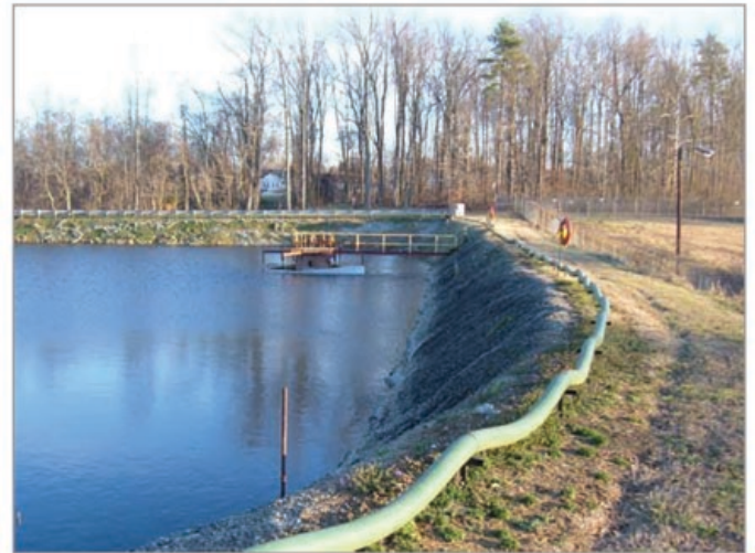
Vapor Distribution Line installed around Lagoon
